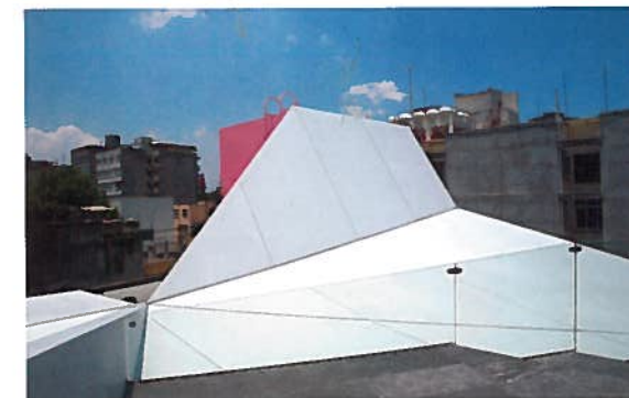
The origamilike form, constructed of Corian, stands in contrast to the surrounding urban landscape.
